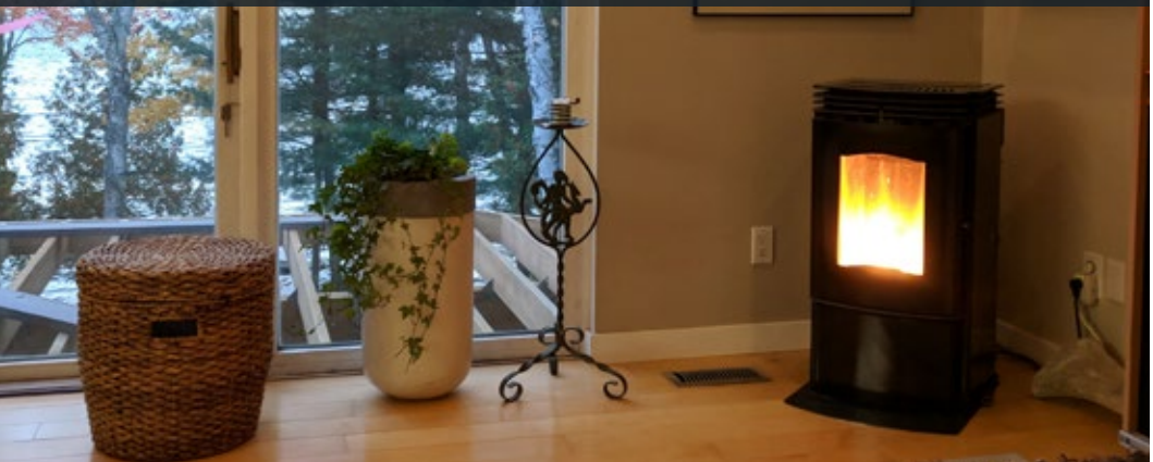
Figure 11. A residential wood pellet stove. Partial bags of pellets are stored in the basket (on the left) until needed. This stove provides heat for most of the year for this typically sized home, using about 200 bags of pellets (3.6 tonnes). (Photo: Innovations Initiatives Ontario North)
