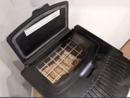
Figure 12. Pellets are loaded into the hopper of the pellet stove, as shown. A control system then automatically moves the pellets to the stove's combustion chamber as required. (Photo: Innovations Initiatives Ontario North)
