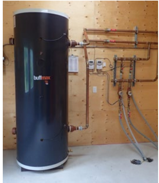
Figure 32. The boiler and pellet hopper (left) feed hot water to the storage tank (right). Hot water is then supplied to Haliburton Solar and Wind and Haliburton Highlands Brewing and is used for space heat and domestic hot water. The energy meters used to bill the businesses can be seen on the wall beside the storage tank.
