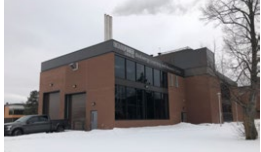
Figure 25. Wood chip boiler room and fuel storage facility at Confederation College. The garage door on the left leads to the on-site wood chip storage room. The door on the right leads to the boiler room. The system can be seen by passersby through the large windows. Wood chip boiler rooms do not need to be this large, but this boiler room was designed to accommodate tours and teaching. (Photo: Biothermic)
