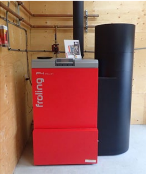
Figure 32. The boiler and pellet hopper (left) feed hot water to the storage tank (right). Hot water is then supplied to Haliburton Solar and Wind and Haliburton Highlands Brewing and is used for space heat and domestic hot water. The energy meters used to bill the businesses can be seen on the wall beside the storage tank.
