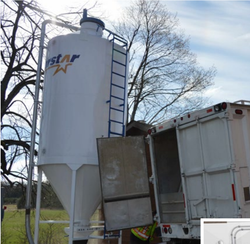
Figure 9. Delivery truck unloading pellets into a water-tight agricultural silo using a vacuum hose. An automatic control system tells the combustion system when to move pellets from the silo to the combustion system. (Photo: Biothermic)
