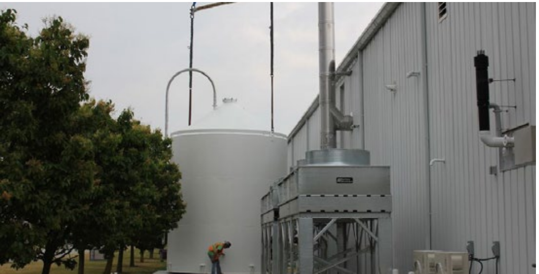
Figure 35. A 35 metric ton silo is used to hold wood pellets at Veissmann's Canadian Headquarters. (Photo: Viessmann Manufacturing Company Inc.)
