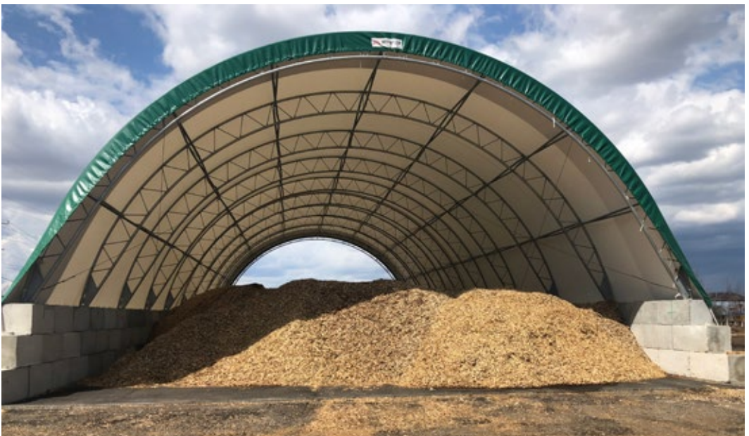
Figure 30. This bioheat wood chip production facility has an asphalt pad to eliminate dirt and sand contamination and keeps the chips covered to allow them to dry. It stores 1 000 oven-dry tonnes. (Photo: Biothermic)
