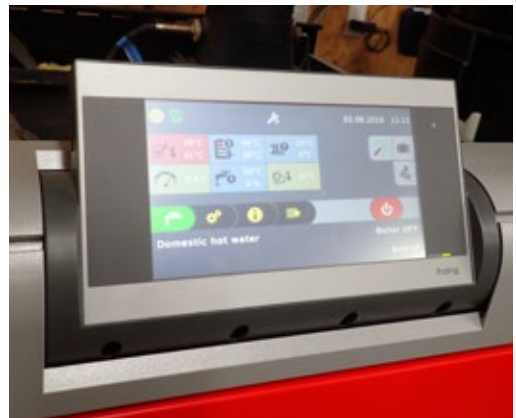
Figure 20. Combustion systems can come with sophisticated controls that manage building temperature levels and schedules and domestic hot water in addition to the combustion system itself. These control systems ensure clean and efficient combustion, monitor fuel levels, and control fuel conveyance systems. This is a control system for a pellet boiler, but it would be similar to other boilers as well.
