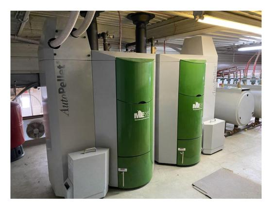
2-56 kW MESys boilers with 2 horizontal buffer tanks
