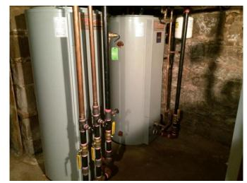
56 kW ÖkoFen boiler with a buffer tank and indirect water heater
