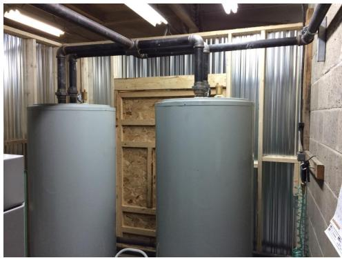
56 kW ÖkoFen boiler with 2 buffer tanks
